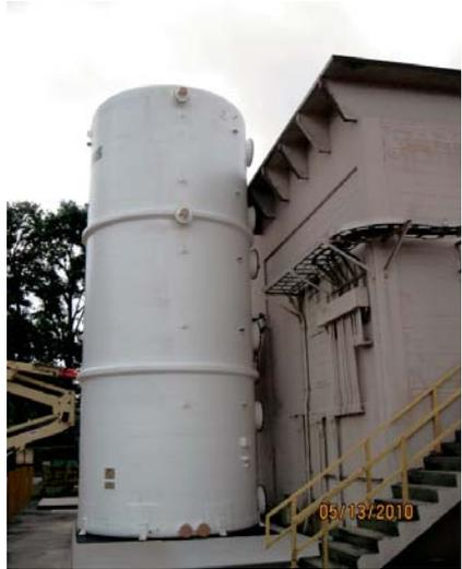
A new biotower unit at the NWWTP will reduce the odors caused by hydrogen sulfide produced in the plant.
