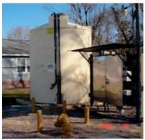
Chemical feed systems installed at five pump stations will reduce odors produced by wastewater.
