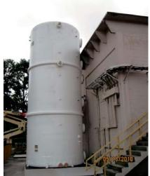
A new biotower unit at the NWWTP will reduce the odors caused by hydrogen sulfide produced in the plant.
