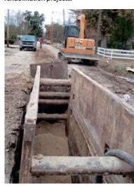
The Elm Grove Garden Road to Harding Boulevard rehabilitation project involved the removal and replacement of sewer pipeline and manholes.
