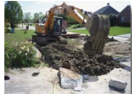
Construction work finished in October in the Azalea Lakes Area.
