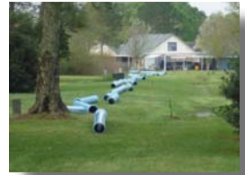
Over 14,500 linear feet of new forcemain was laid in the Gurney-Joor area. Construction completed in November 2009.
