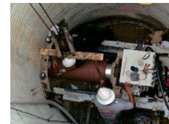
MTBM is pushing 12" heavy-wall clay pipe.
