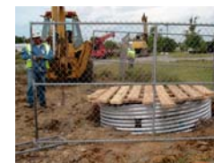
120-inch diameter CMP tunnel shaft is augered into the ground to a pre-determined depth at the RMAP1-Industripex Project. At night the area is secured for safety.
