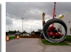
120-inch diameter CMP tunnel shaft is augered into the ground to a pre-determined depth at the RMAP1-Industripex Project. At night the area is secured for safety.
