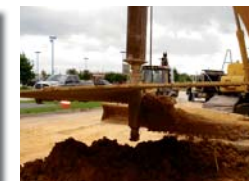
126-inch diameter auger bit used to create the hole that the corrugated metal pipe (CMP) will be placed.
