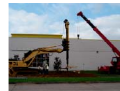
126-inch diameter auger bit used to create the hole that the corrugated metal pipe (CMP) will be placed.
