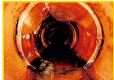
As part of the CCTV inspection, sewer lines and manholes will be cleaned of blockages and debris. Any fractures will be identified and reported for repair evaluations.
