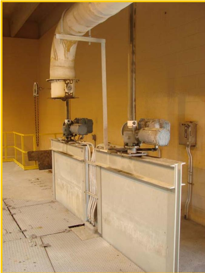
This system will address odor problems in the collection system and will result in a reduction in odor at the receiving treatment plant.
