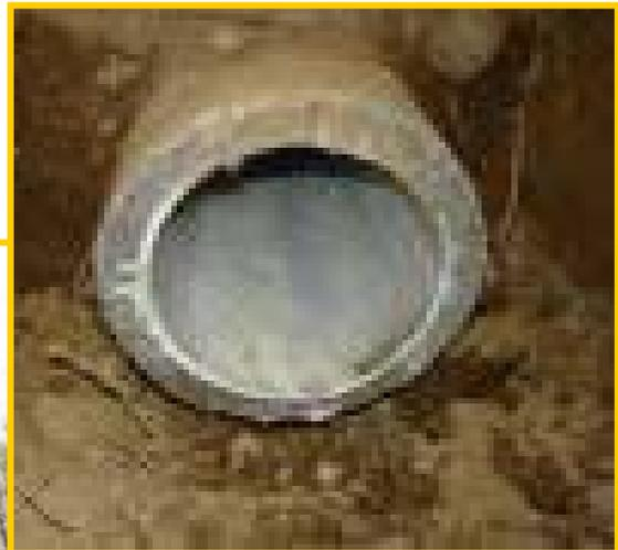
A typical gravity pipeline after cleaning and CIPP.
