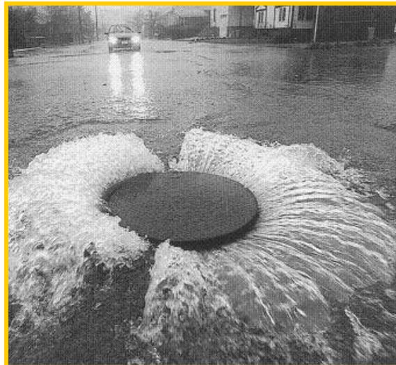
Manholes are a large source of inflow and infiltration (I&I) into sanitary sewer systems. Inspection and repair is one of the most cost effective means of reducing overflows.
