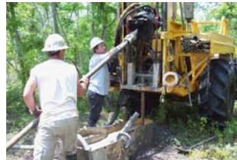
Geotechnical investigations were conducted at the SWWTP.
