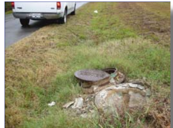
775 manholes will be inspected in the Scotland Avenue – Progress Road Area.
