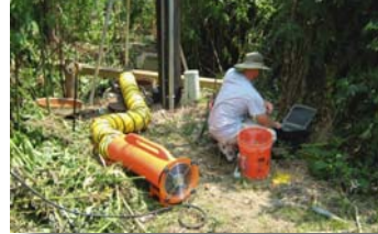
168,300 linear feet of pipe is inspected in the Gardere – Burbank area.
