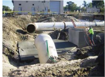
Construction of yard pipe at the SWWTP that will convey wastewater throughout the plant.
