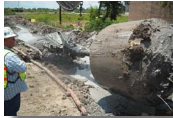
Horizontal-Directional Drilling in the Staring Lane Extension area.
