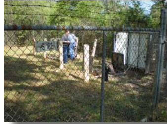
As part of the Group 2 Project, Pump Station # 182 located near YMCA Drive will be replaced.
