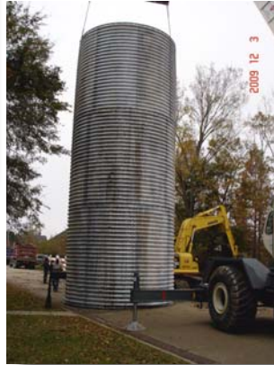
A 14" diameter wet well casing is being installed at Pump Station 134.
