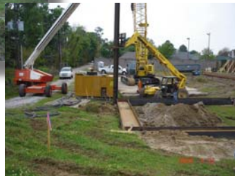
Installation of a 24' foot deep coffer dam in preparation of construction inside Pump Station 136, near Sherwood Forest Boulevard.
