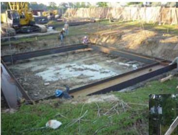
Installation of a 24' foot deep coffer dam in preparation of construction inside Pump Station 136, near Sherwood Forest Boulevard.
