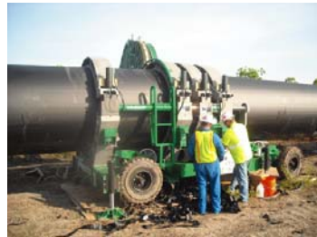
A fusing process is used to join two segments of the 65" HDPE pipe together.
