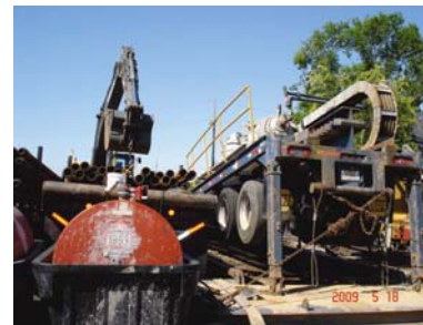
Construction crews mobilizing drill rod equipment that will be used for the HDD pipe installation in the Staring Lane area.
