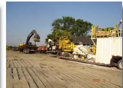
Construction crews mobilizing drill rod equipment that will be used for the HDD pipe installation in the Staring Lane area.
