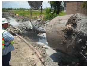
Completing the first of two Horizontal Directional Drills
